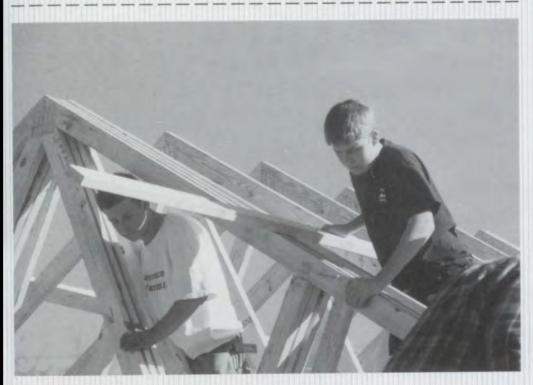
Working on the job site, a.m. building trades students Jesse Schaefer and Chris Faulkenburg arrange heavy trusses for the framing of the house. The two building trades classes work at the site every day. technical skills such as plumbing, roofing and masonry work.
