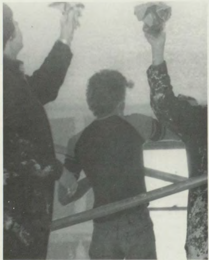
Above: The construction of playground equipment is no easy task, as shown by Barry Hammack and Scott Pannett.
