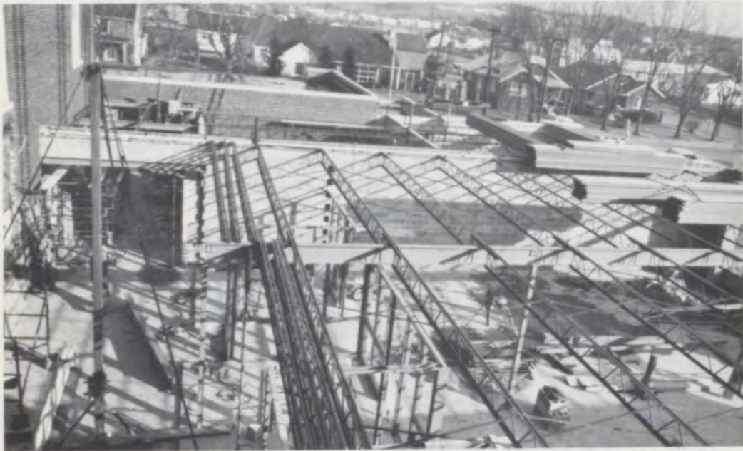
PROGRESS OF OUR NEW ADDITION, FALL AND WINTER OF 1962-1963.
