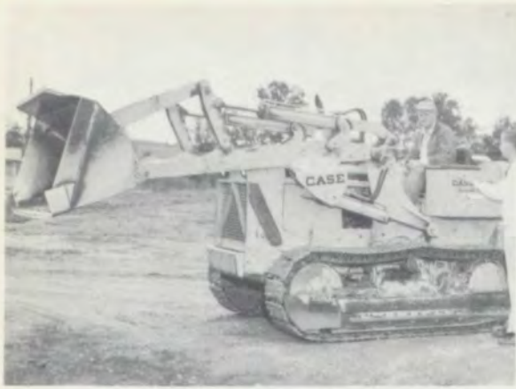
Richard Wheatly has learned that HERMAN PETERS is tops when it comes to excavation and building.
