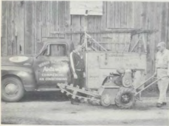
Leroy Neyenhaus thinks Mr. Huebschman's plumbing devices are just grand.
