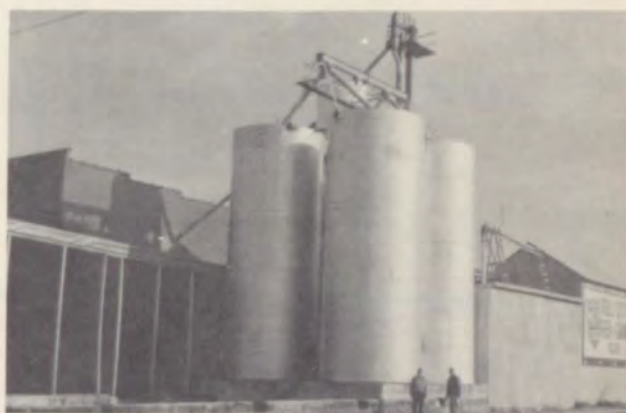
The brand new grain elevators at the TELL CITY FLOURING MILL are being carefully appraised by Martin Harpenau.
