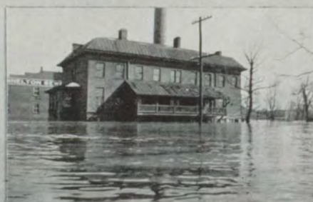
Sewer Pipe Office
